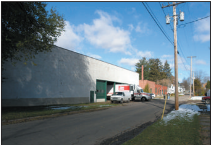
Fig. 9 When I visited, they were just getting things set up in the new facility and the rigors of running two different locations were evident.
