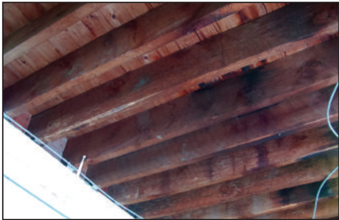
Fig. 9. The building was originally built as a car dealership and showroom with the appropriate construction to support the weight.
